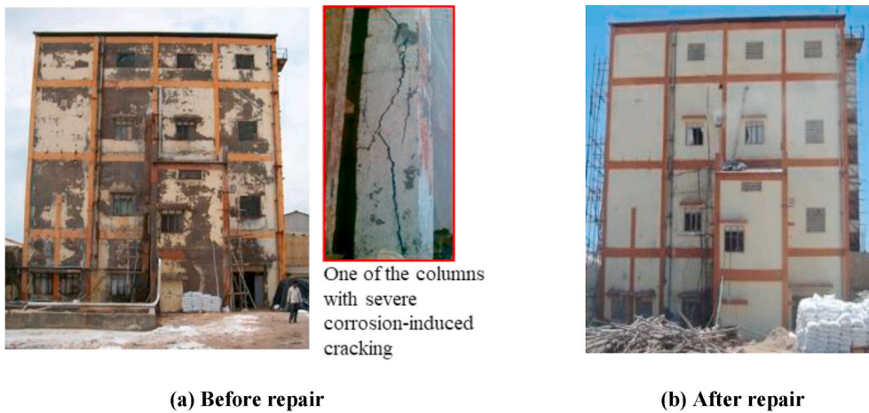
Fig. 10. Industrial building (salt processing unit) before and after the repair in 2008.
